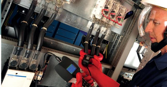
Our experts go on site and help you to check the functioning of the Insulation Monitoring Device (IMD), to measure the insulation of your installation and to detect and localize faults up to the end feeders/lines.
